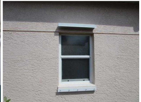
most glazed openings are protected
