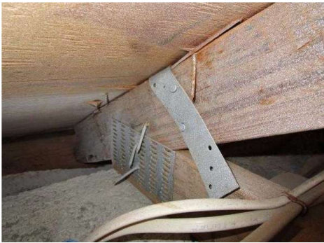
8d nails spaced no more than 6 inches apart
